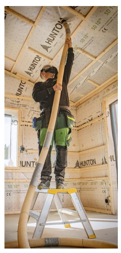
Blown-in insulation of Nativo Wood Fiber Insulation is a fast and efficient insulation solution for all types of buildings. By using Nativo Wood Fiber Insulation Blown-in, carpenters save valuable work time. For example, in an open attic, we can insulate up to 1000 m² per day. This is about twice as fast as using boards.
